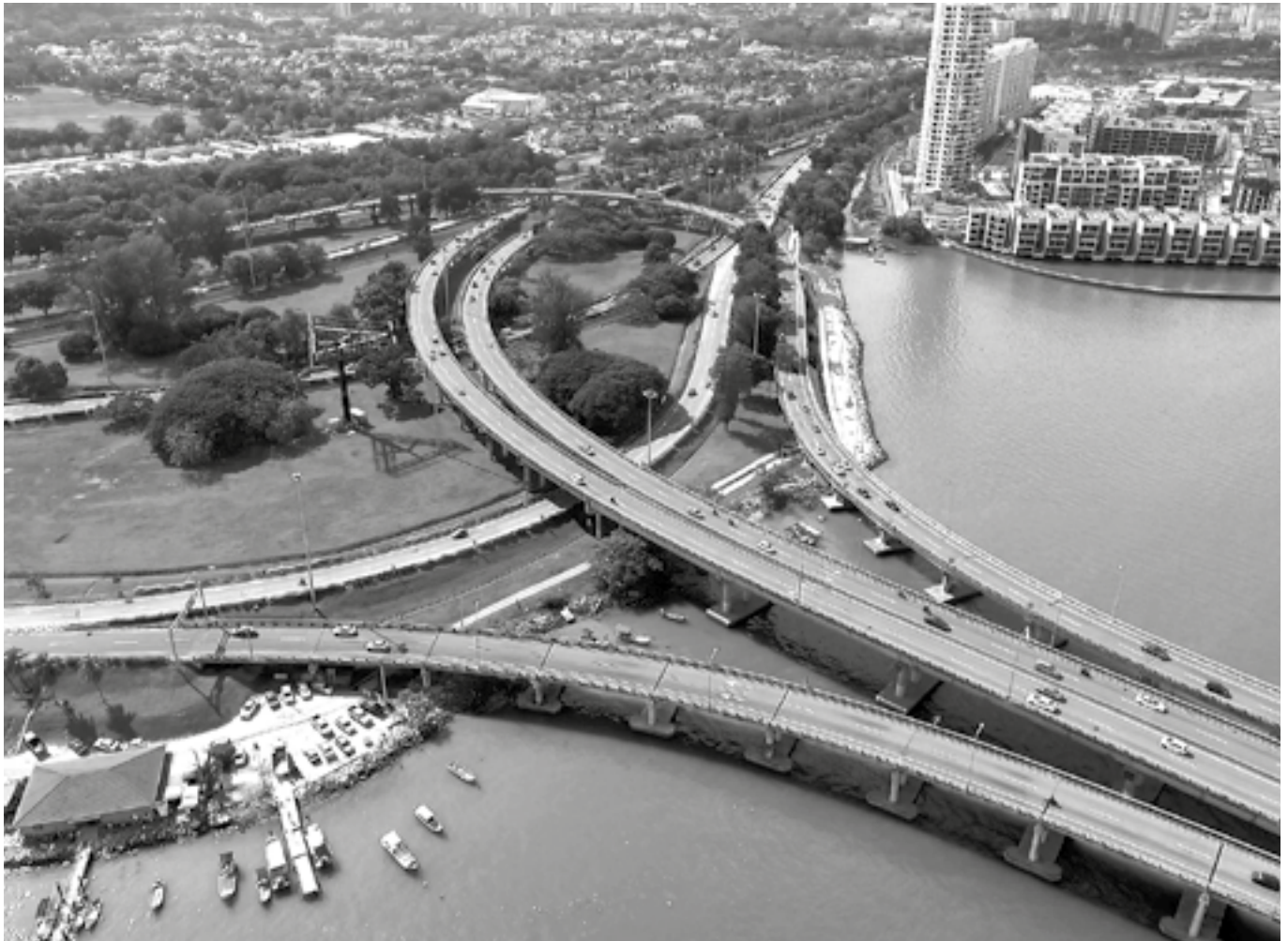
Penang Bridge widening
