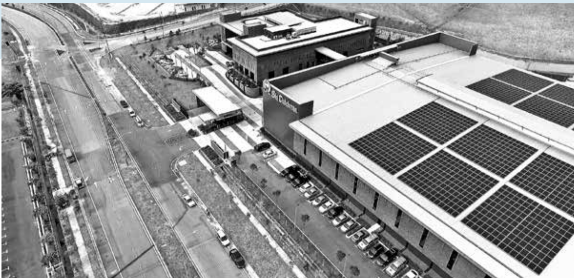
Big Dutchman - Warehouse and Office Building
